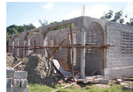
Fosse Capois school under construction
