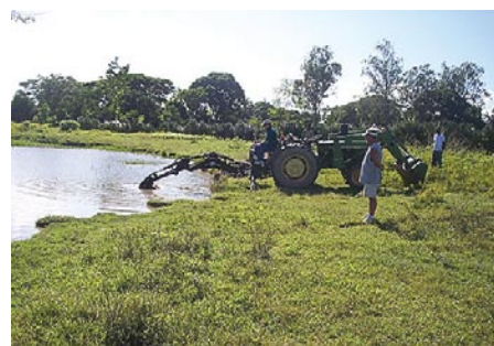
Fishpond in progress
