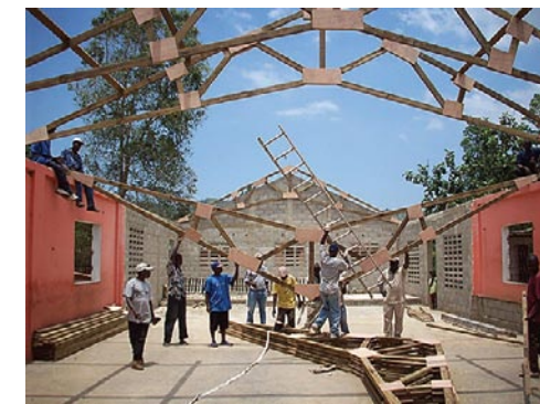
Haitian crew works on addition in Juchereau
